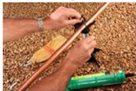
Only one nylon tie is necessary to secure pipe to Pipe Prop.
